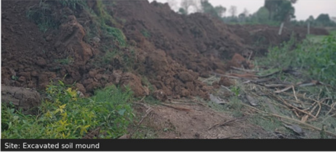
Site: Excavated soil mound
